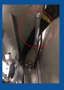
Step 7. Lift the car sling slightly off the ground with the hand crank, and then tighten the bolts
