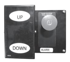
**Step 3:** Press and hold the UP rocker. The lift will move in the up direction and stop when it reaches the upper landing.
