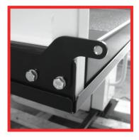
**Step 3:** Attach the ramp to the pivot tabs using shoulder bolts and locking nuts. Tighten the nuts until they seat against the bolt shoulder.
