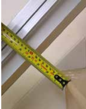
RAIL TO STEP NOSE MINIMUM OF 3 1/4"
