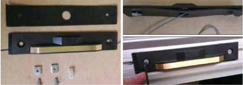
The charge/end stop assembly determines the height of the stairlift finishing position at the bottom of the stairs. The assembly must be at least 70mm (2 3/4") from the end of the rail. Fit rail end cap.
