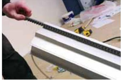
Unpack Drive Unit. Load at top of track carefully. Ensure that lower carriage rollers are located into rail extrusion channels correctly and that drive and OSG pinions do not catch. Lower Drive Unit, slowly down the Rail Extrusion until drive pinion rests against lower rack section. Do not install top section of gear rail until carriage is loaded on rail.
