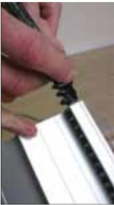
Mark racking flush with rail extrusion, remove and cut ensuring cut is level. Slide racking back into position. Ensure that cut section of rack is at the top of the rail. Fit top end stop / charge assembly. Again, the position of this sets the stairlift height but must be at least 55mm from end of rail. Coil any spare cable and push into top of rail.
