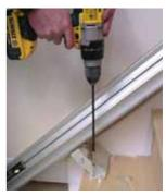
Screw down rail and tighten all leg bolts allowing for thickness of step covering to maintain the minimum step clearance distance. Ensure that each foot in attached using 4 screws supplied.
